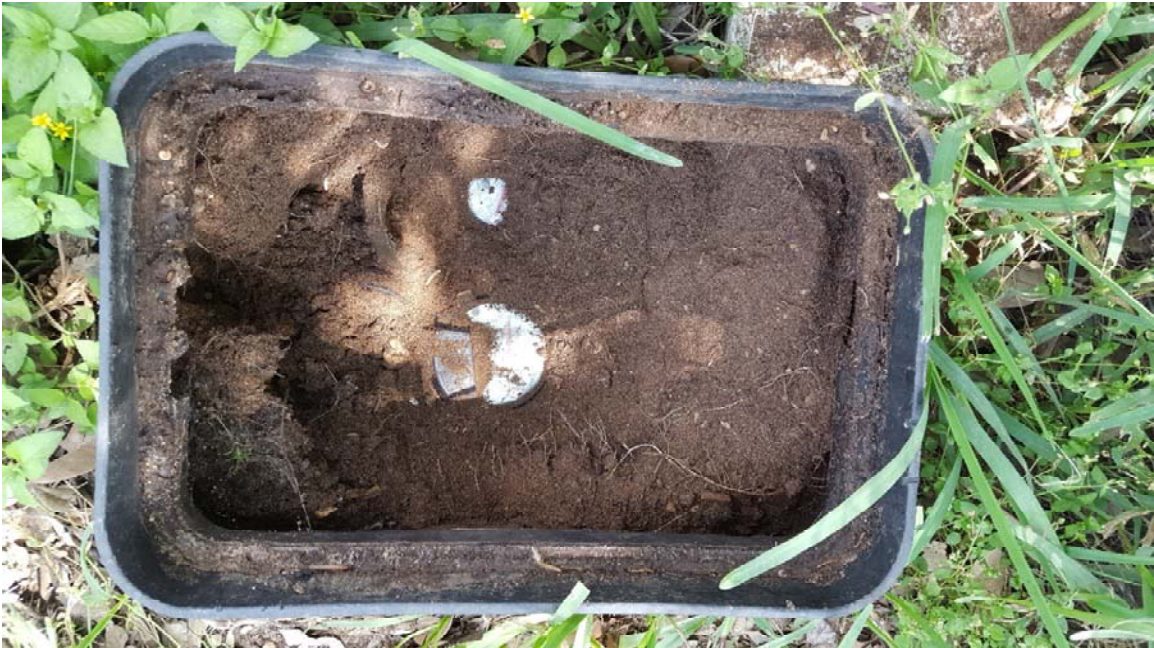
Photo 6 – Cycle 16 Meter at 145 Timbercreek Rd (2 meters in same box; return to SAWS)
